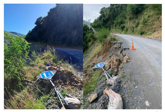
The picture on the left is from the 5<sup>th</sup> of April 2023 and the photo on the right is from the 9<sup>th</sup> of April. There has been a loss of a little more of the road and cracks are present which suggest that further losses of width may shortly occur.
