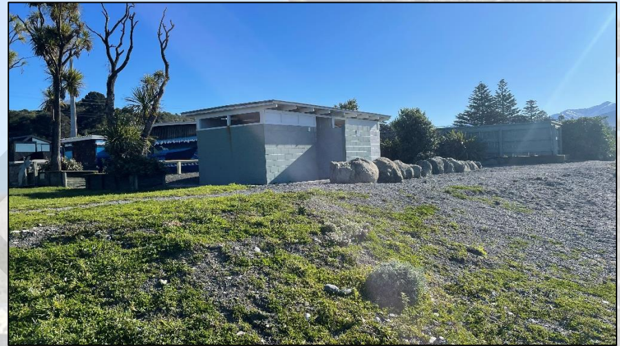
The current toilet and changing room facility from the beach/coastal environment
