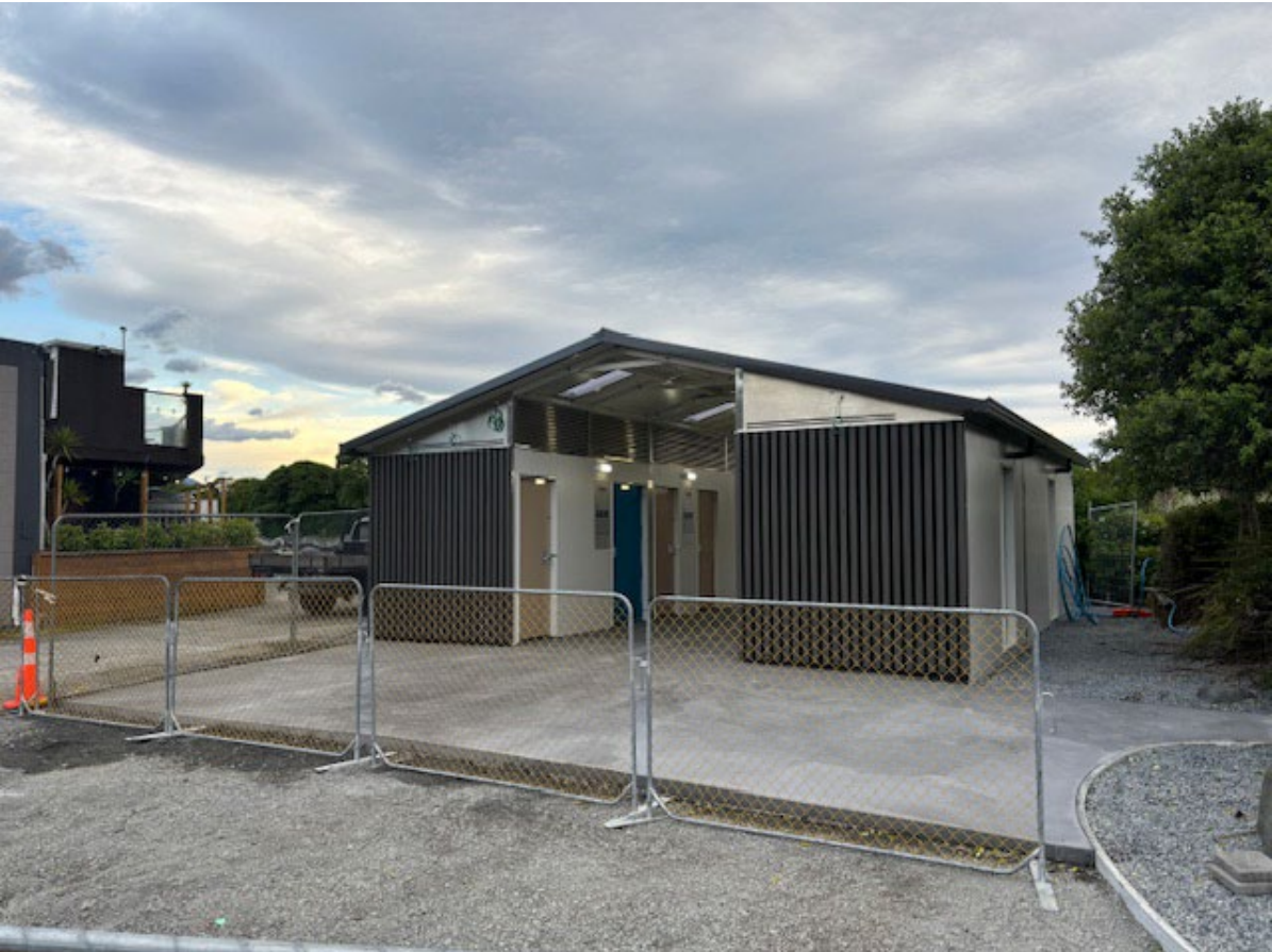
West end toilets
