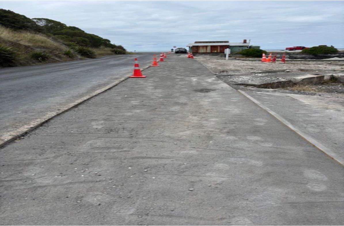
Fyffe quay link pathway surface preparation.
