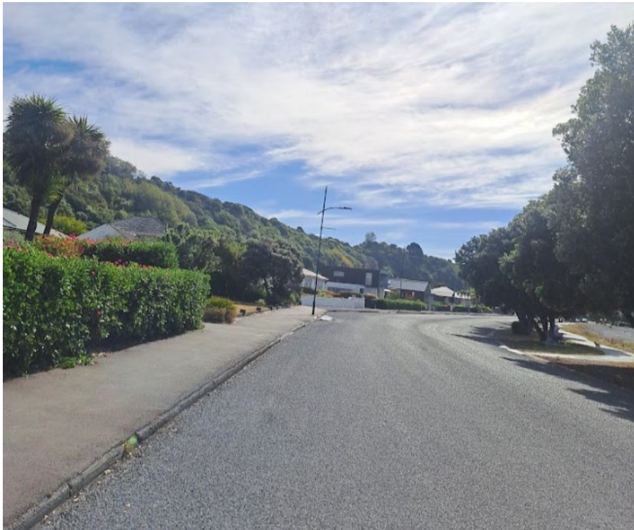
Photo 1: Resurface completed on Esplanade Road
