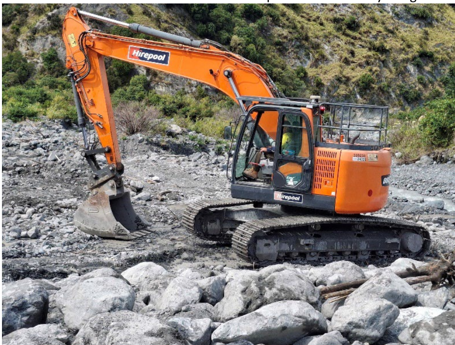
Photo 2: Repairs done in Jordan Stream Ford crossing
