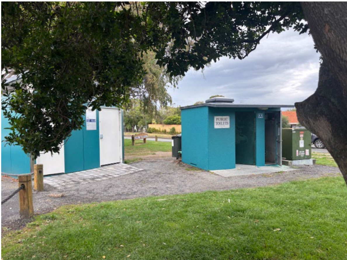
Photo 5: Toilet block at the Top End
